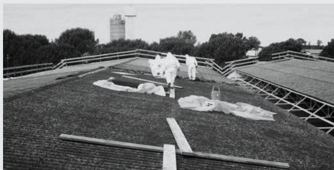
Asbestos removal
