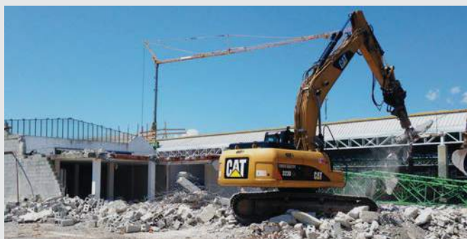
Demolition of old premises
